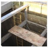
If cages aren't close to the side walls they can be repositioned with upright guide rods. The upper edge of the guide rod has to be above the water level or at least visible after lowering the water level (example Komárno).
