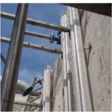
Cross bars at the side walls that support the repositioning of cages in small tanks (example Lahnstein)
