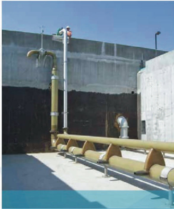
JET MANIFOLD AERATOR
